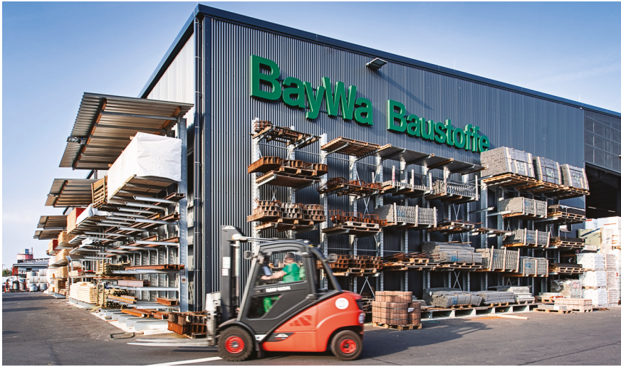
BayWa open-air warehouse for building materials in Großwallstadt
