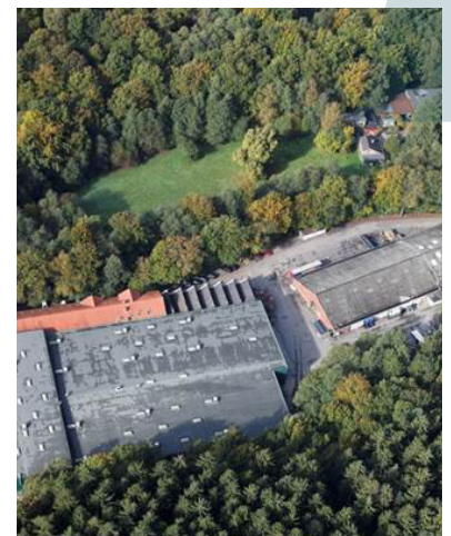
Kabelwerk Eupen AG is one of the largest employers in East Belgium.
